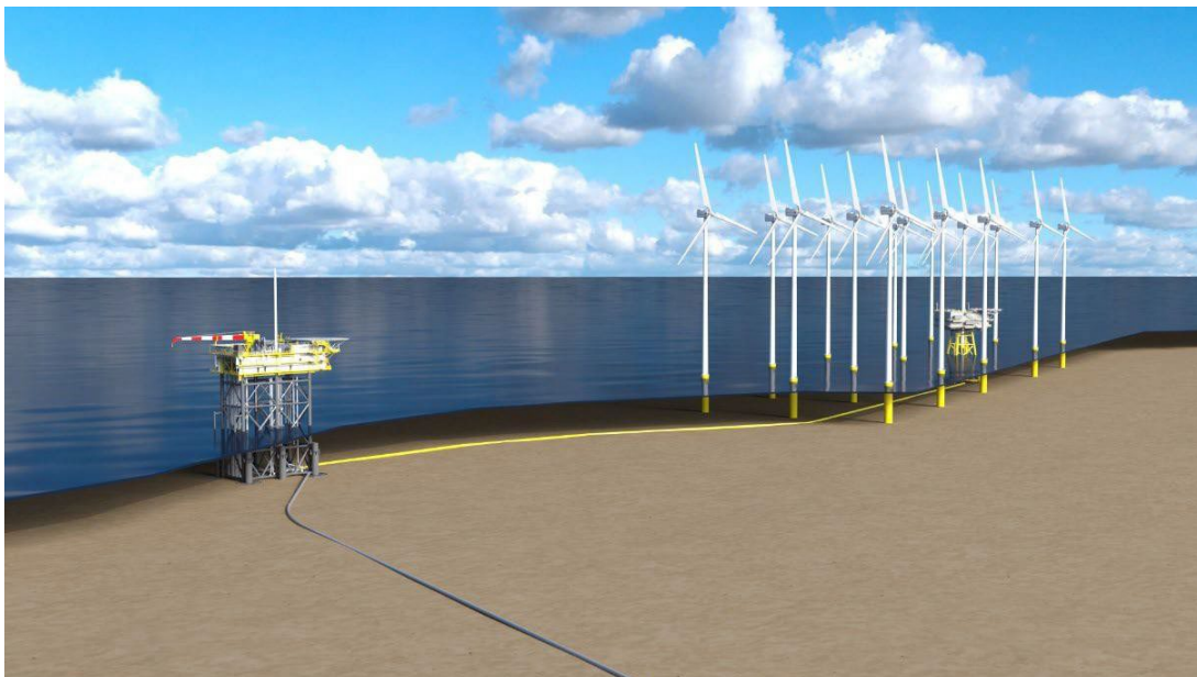
Visualisation of the N05-A platform and the connection to the Riffgat wind park
